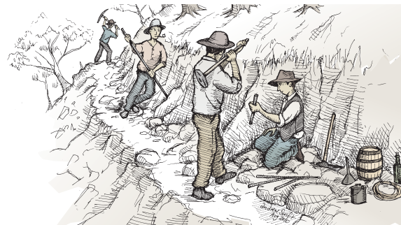
Construction workers preparing rock for blasting on the ditch (A Swift)
